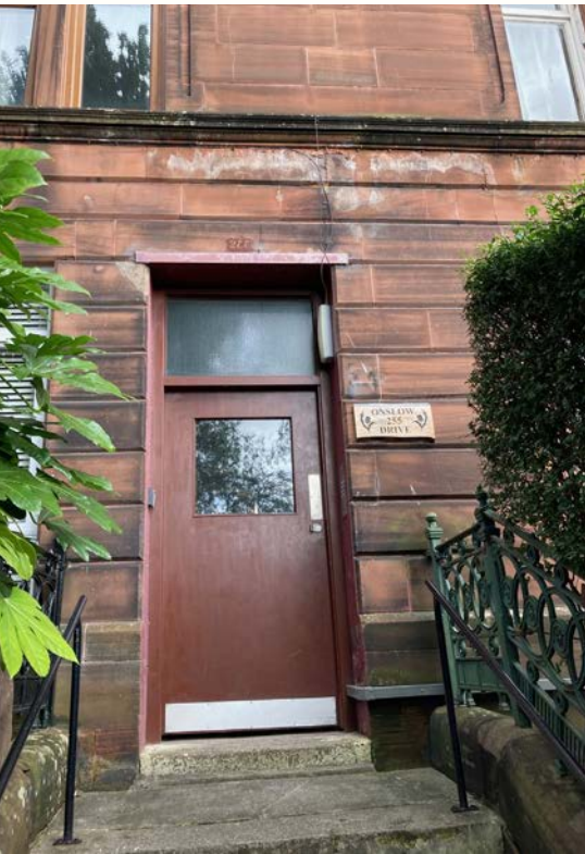
255 Onslow Drive, where the Mullan/Conway family lived, as it is today | Credit: GWL
